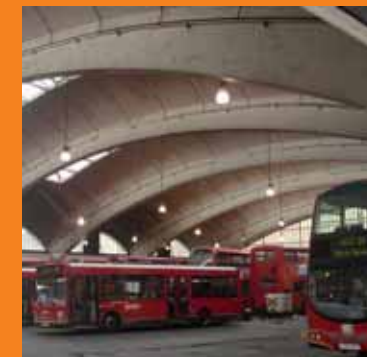
Stockwell Garage Interior
